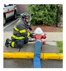
The firefighter "makes up" the hydrant by connecting the LDH (or 4-way valve) to the steamer connection and attaching one or two gate valves to the  $2\frac{1}{2}$ " discharges.
