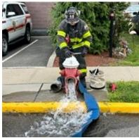
The firefighter removes the steamer cap and opens the hydrant to confirm it is a working hydrant and to flush any debris from the barrel of the hydrant.
