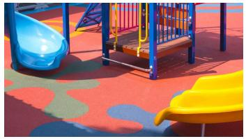
Playground owners wishing to install a unitary material as a playground surface should request ASTMF1292 test data from the manufacturer, identifying the critical height rating of the desired surface. In addition, site requirements should be obtained from the manufacturer because some unitary materials require installation over a hard surface while others do not.
